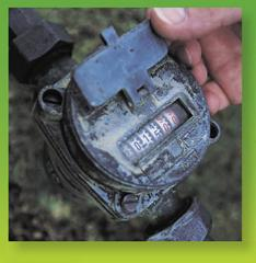
Smaller pipes bring water from the reservoirs, passing through a water meter at the front of every property to measure the water used. Each household pays according to how much they use.
