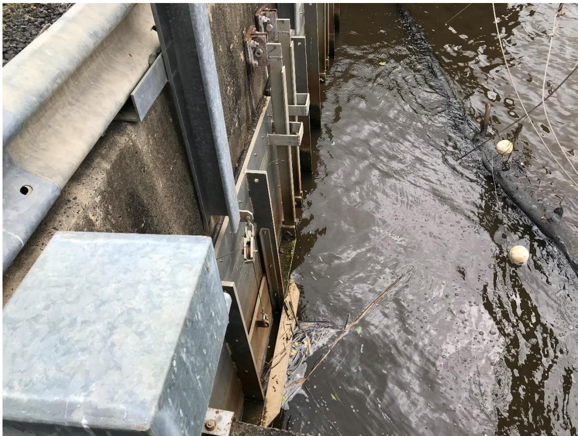
3: Sluice window installed on the floodgates at North Woodburn-Kilgin drain.
