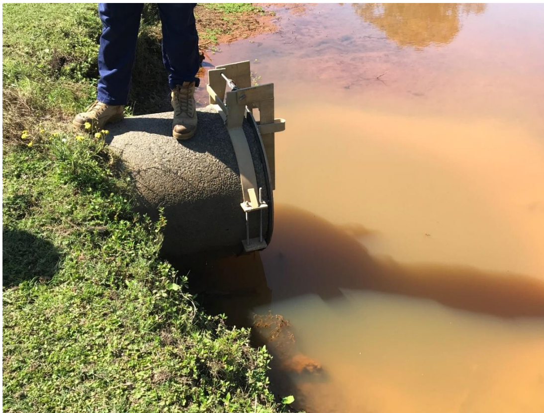
14: An example of the secondary pipes and floodgates installed along Dungarubba Canal, note the abundant flocculated iron in the drain water from acid sulfate soils.
