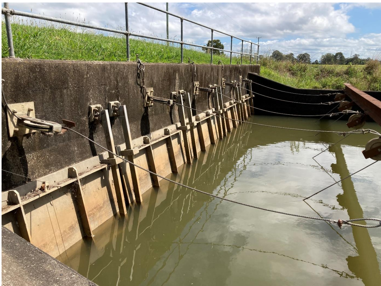
2: Dungarubba Canal floodgates and headwork structure.
