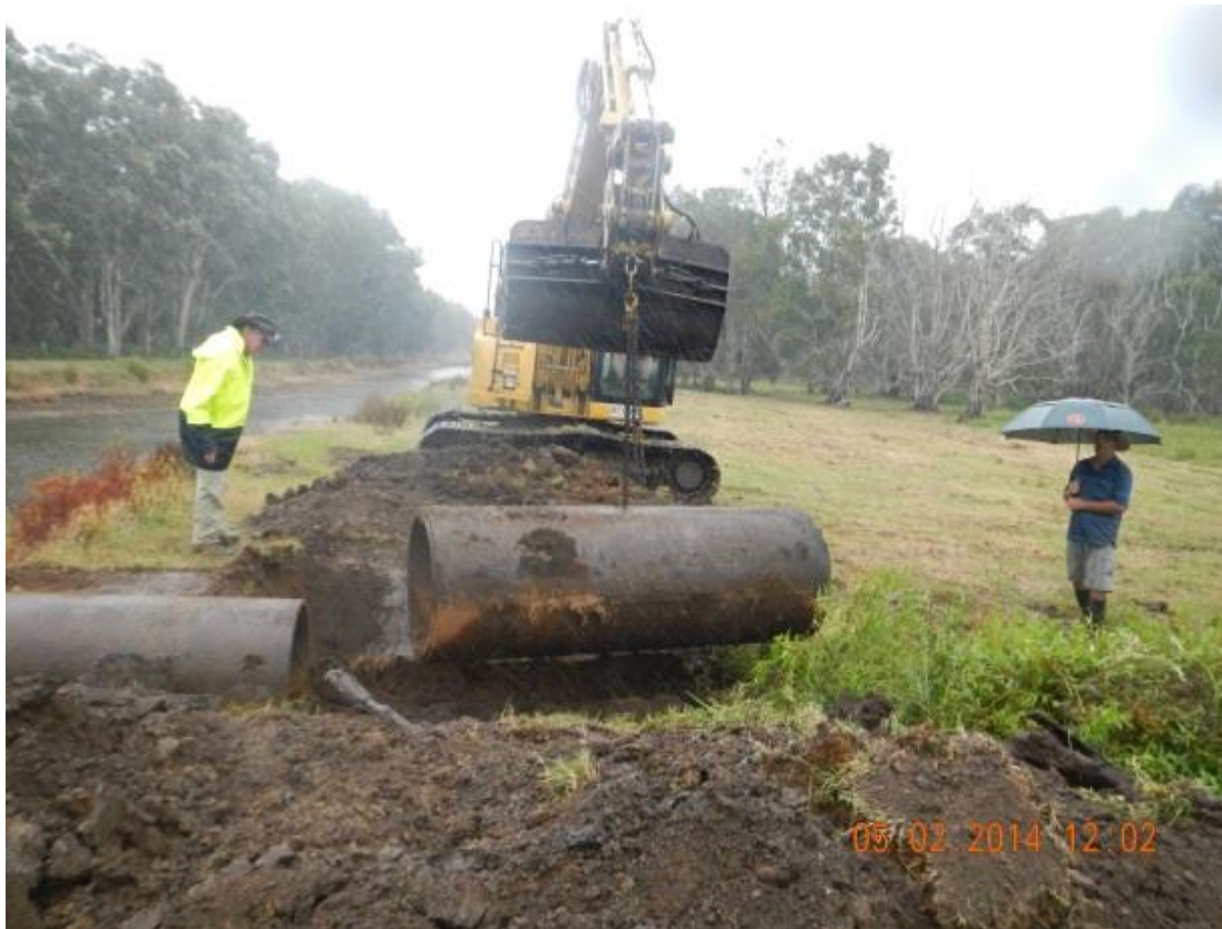
13: Secondary pipes and floodgates being installed in 2014 to restrict tidal water to the main canal.
