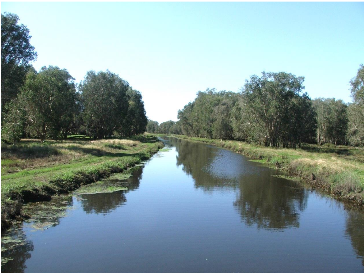
4: Dungarubba Canal as it travels through the lowest lying section, approximately 3 kilometres upstream from the floodgates, note the low bank heights in relation to the drain water level.
