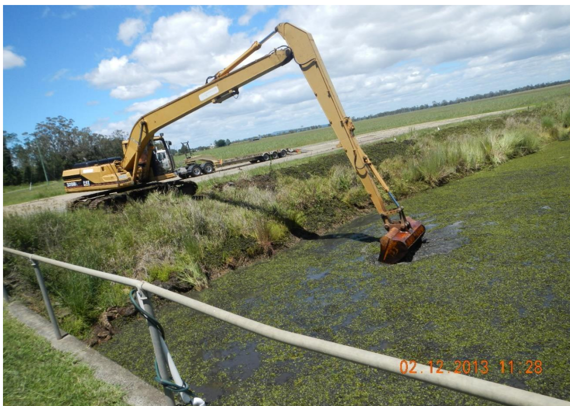
6: Council removing a build-up of vegetation from behind the floodgates.
