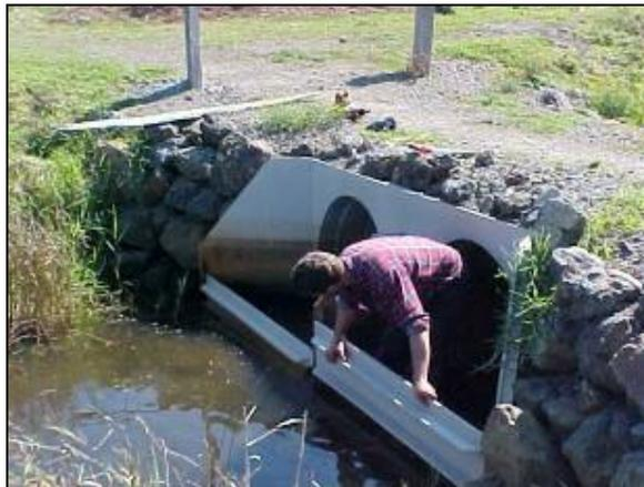
**Figure 6:** *Fitting drop-board culvert to maintain low groundwater gradient (DPI).*
