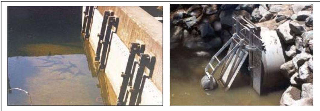
*Figure 17 & 18: Floodgate obstructing fish passage (Scott Johnston, DPI); Automatic tidal floodgates where floating mechanism closes gate.*
