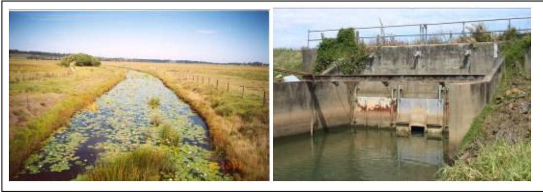
*Figure 15 & 16: Drain clogged with macrophytes; Floodgate structure open to allow flushing and fish passage (DPI).*
