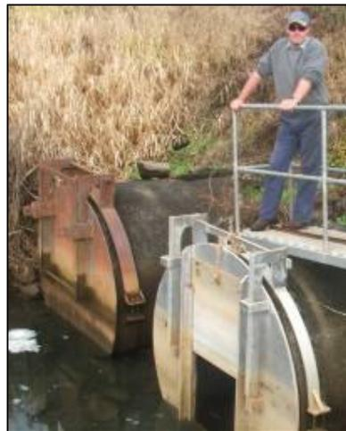
*Figure 19: Floodgate management in action - Reardon's Canal Swan Bay (M. Wood, RRCC)*
