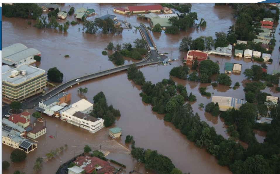
Floodwater flows out of the Wilson River and over the levee wall at the pump station (bottom, centre) on Molesworth Street, Lismore. Picture: Rotorwing Helicopters.
