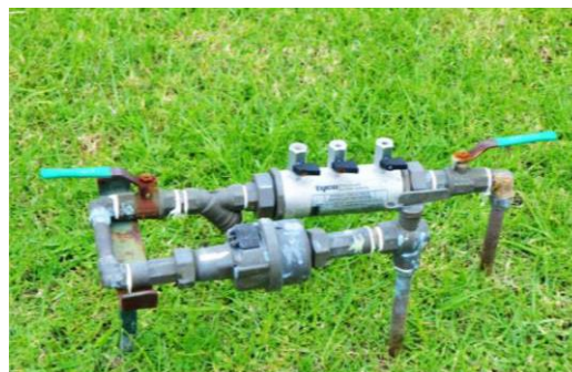
20mm water meter and double-check valve.
