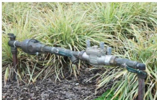
32mm water meter and RPZ device.
