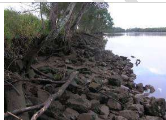
Bank slumping and rock retainment.
