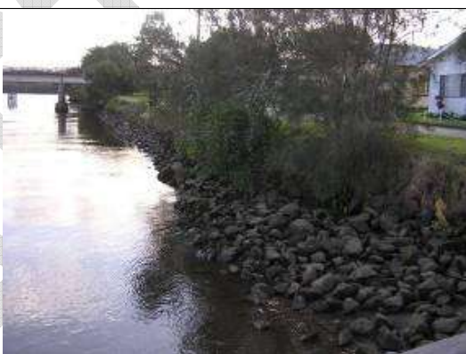
Erosion control at Wardell
